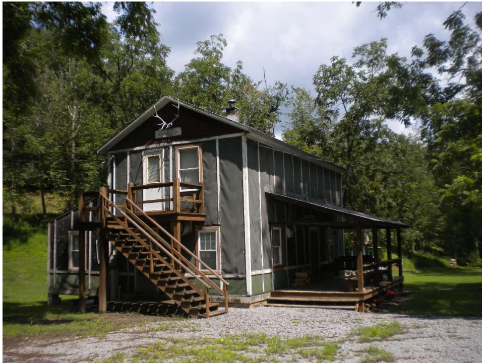
The dormitory at Camp Luey, able to accommodate 75 campers. picture taken August 2021
