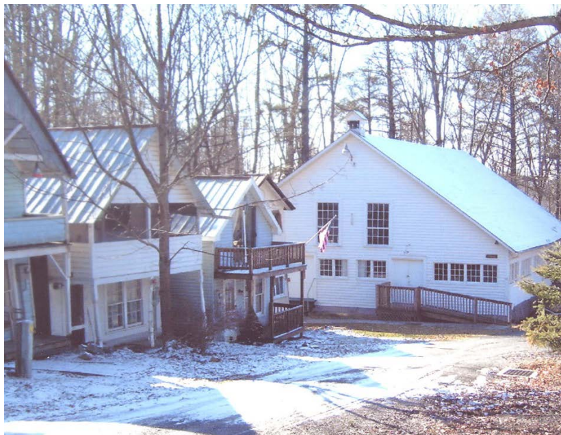
Dimock Camp Meeting cottages and chapel, 2012 Dimock Township, Susquehanna County
