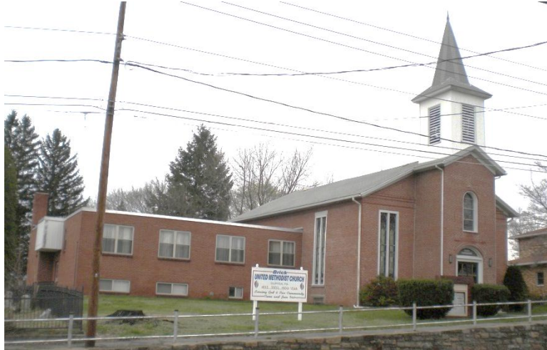
Brick United Methodist Church Duryea Borough, Luzerne County
