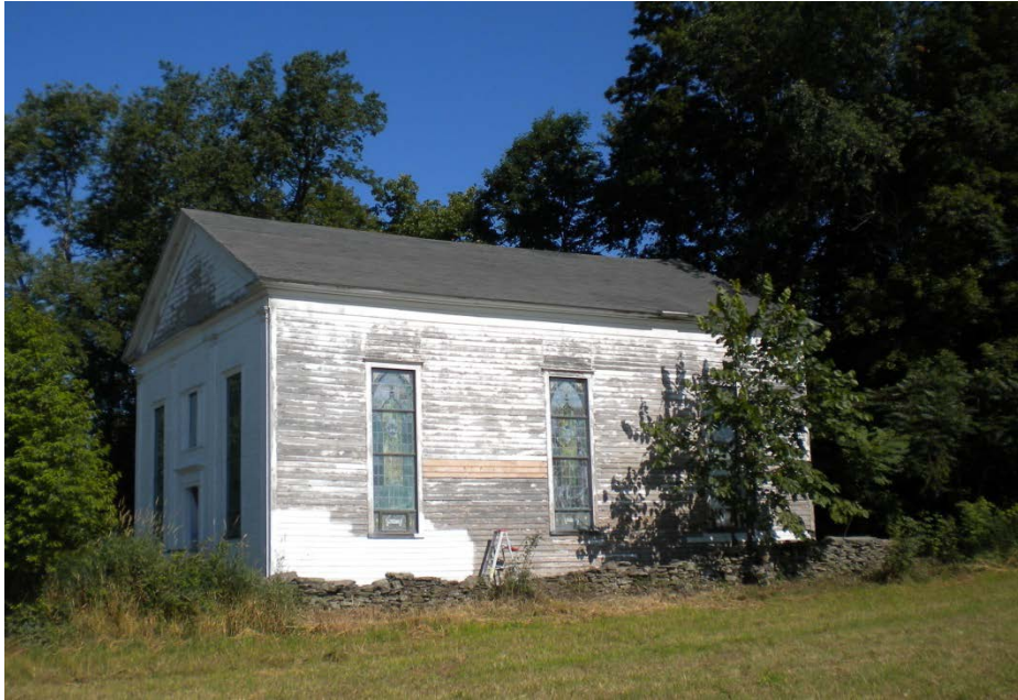
Lymanville Church, while being restored in 2010 Springville Township, Susquehanna County
