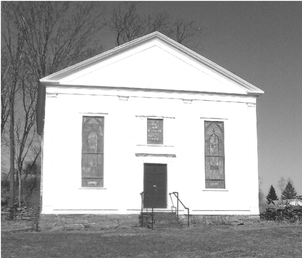
fully restored Lymanville Chapel, 2012
