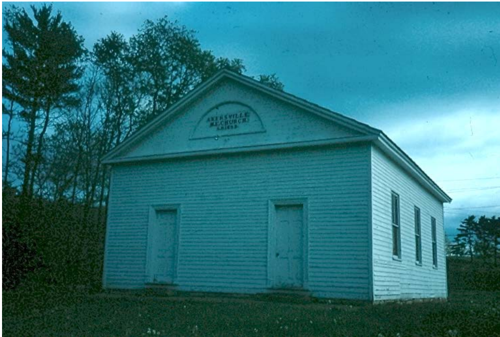
Akersville Methodist Church erected 1858 – dismantled 2015 served by James D. Mathews 1911-13
